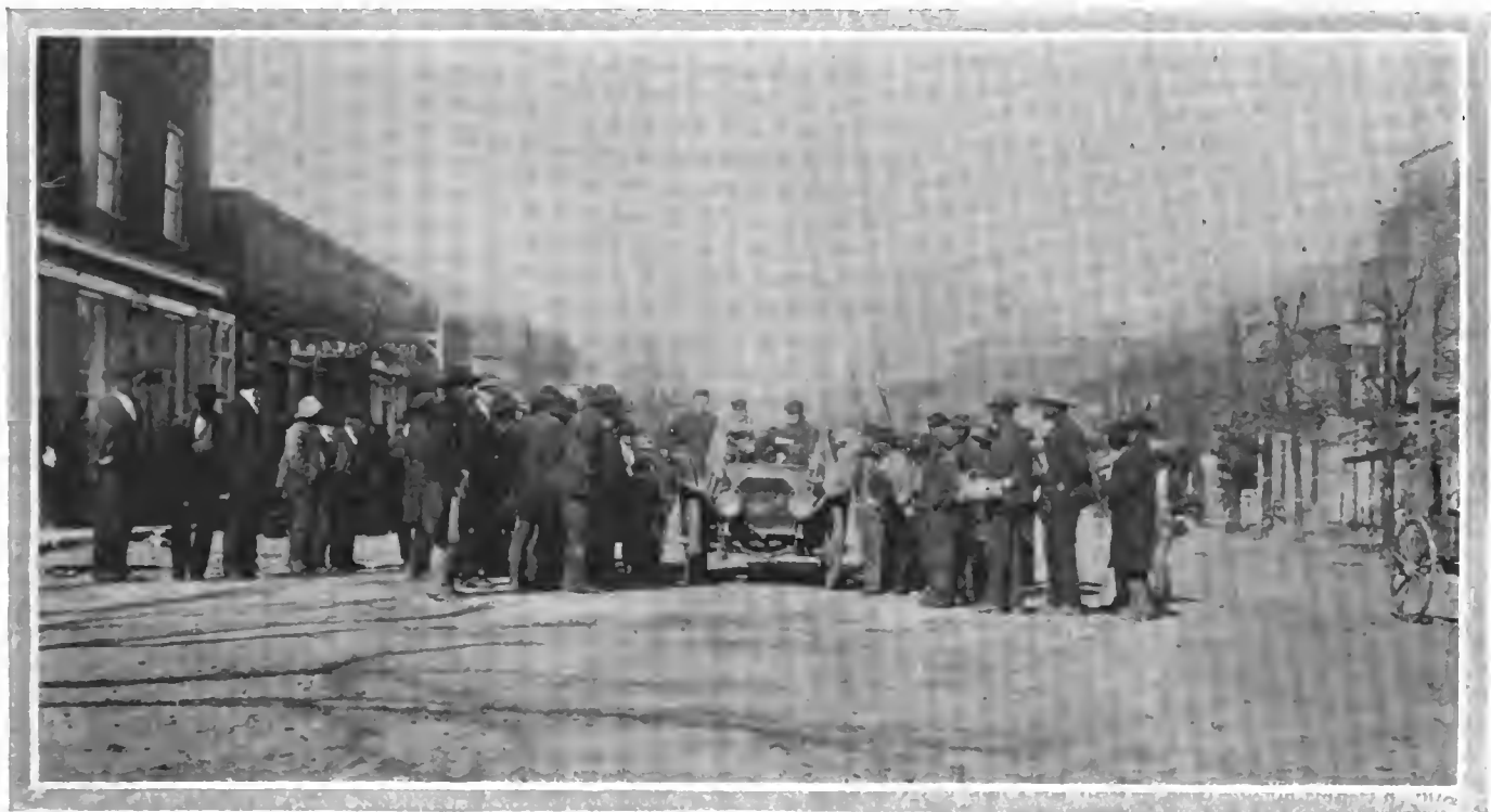
THE PATHFINDING "ALLIGATOR" ATTRACTED ATTENTION ALONG THE ROUTE. THIS PICTURE IN WINNSBORO, S. C., BEING TYPICAL.
